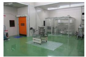
This work space is filled with air that has passed through a high-performance filter,
